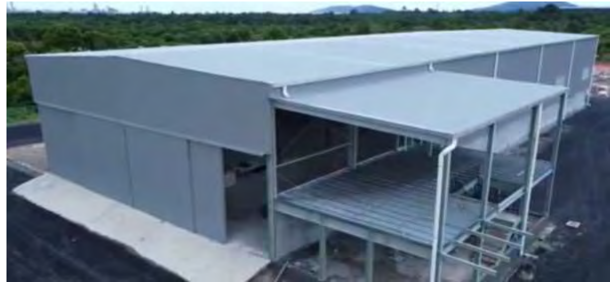
New Workshop at Pengerang, Johor.
